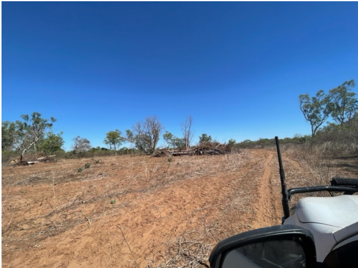
Figure 5. Pump site clearing images - 1 August 2023
